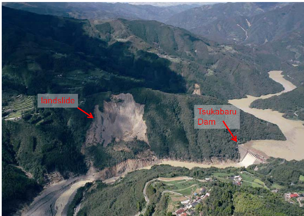
Photo 2 Typical landslide developed near Tsukabaru Dam, Mimigawa River (Miyazaki Prefecture, September 2005).
